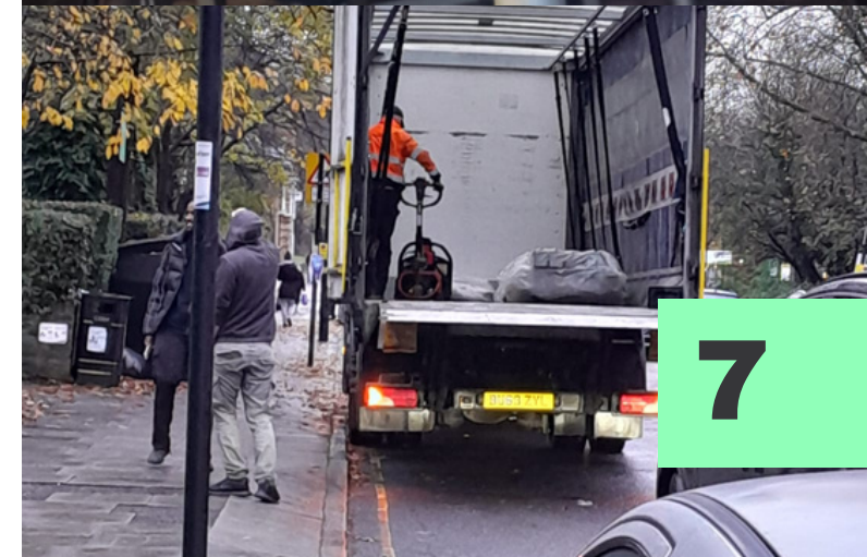
Top: pilot core hole being drilled for MVHR unit Bottom: offloading of equipment
